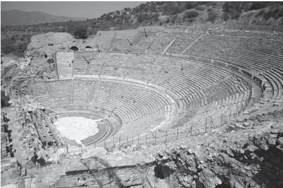
Figure 3. View to the auditorium from south. The arrows show the change of construction technique in the substructure of the seating areas: larger-sized blocks in the area of the slope and opus caementitium outside of it (Irmengard Mayer).
