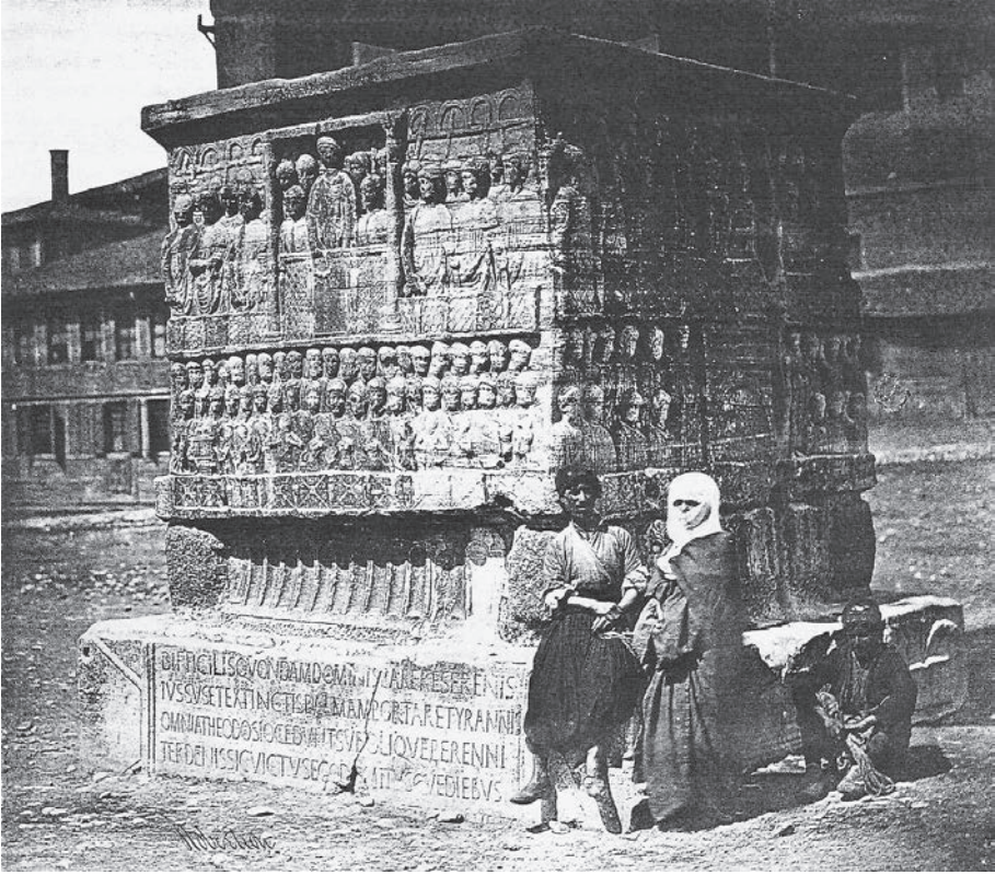
Figure 2. Base of the ancient Obelisk photographed in 1854 by James Robertson, when it was accessible before being framed with iron balusters (Öztuncay, 2003, 121, authorized for publication by Öztuncay).
