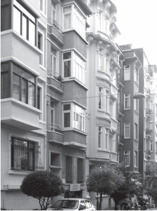
Figure 6. Apartment houses built during the first stage of Turkish Republic within Istanbul Cihangir district (Emiliano Bugatti).
