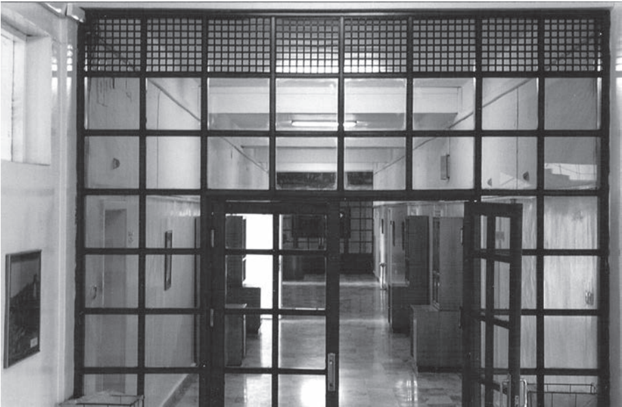
Figure 7. B. Taut, Faculty of Letters and Geography, Ankara 1937 – '39, the dividing wooden and glass screen between the classrooms and the professors' offices, (Paola Ardizzola, 2001).
