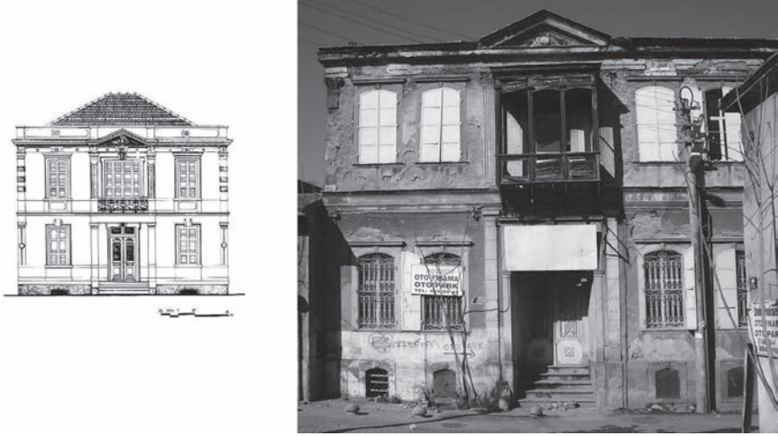
Figure 4. On the left a suburban house in Salonica and on the right a single family house in İzmir Basmane district (Anthologia Ellenikes arhitektonikes, 1981 and picture by Emiliano Bugatti).
