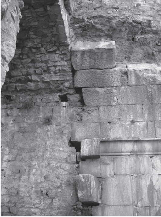
Figure 5. Barrel vaulting in the southern vomitorium to the first diazoma . The in situ “waiting blocks” of a shielding wall show the junction between the high and low vaulting (Gudrun Styhler-Aydin).
