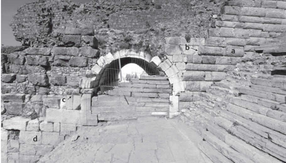
Figure 6. South façade of the theatre with the entrance to the central diazoma (Irmengard Mayer). a) Façade made of local grey marble blocks, the fronts of which have a cushion form b) Starting point of the new wall section, dated to 102-112 A.D c) Detail of wall division d) New wall section made of light blocks in whitish yellow colour with a smooth appearance.
